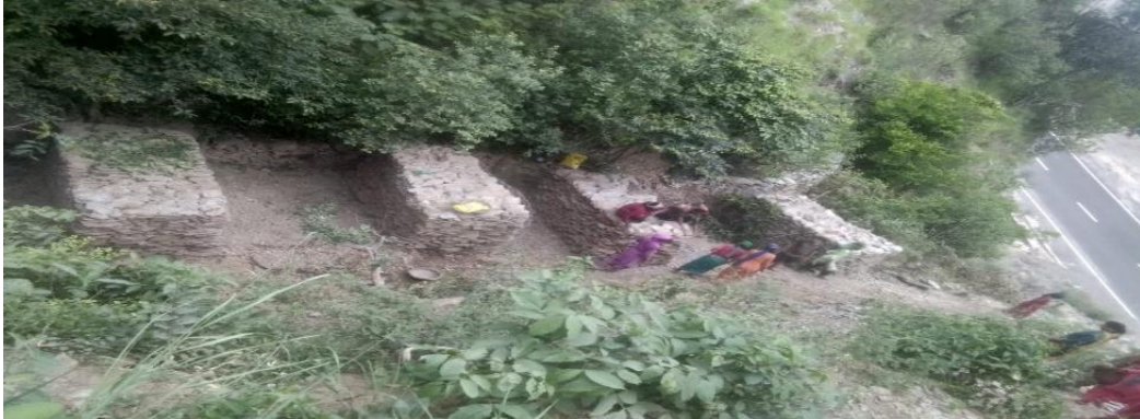
Stone crate wire Gabion structure-Muliyagaon
